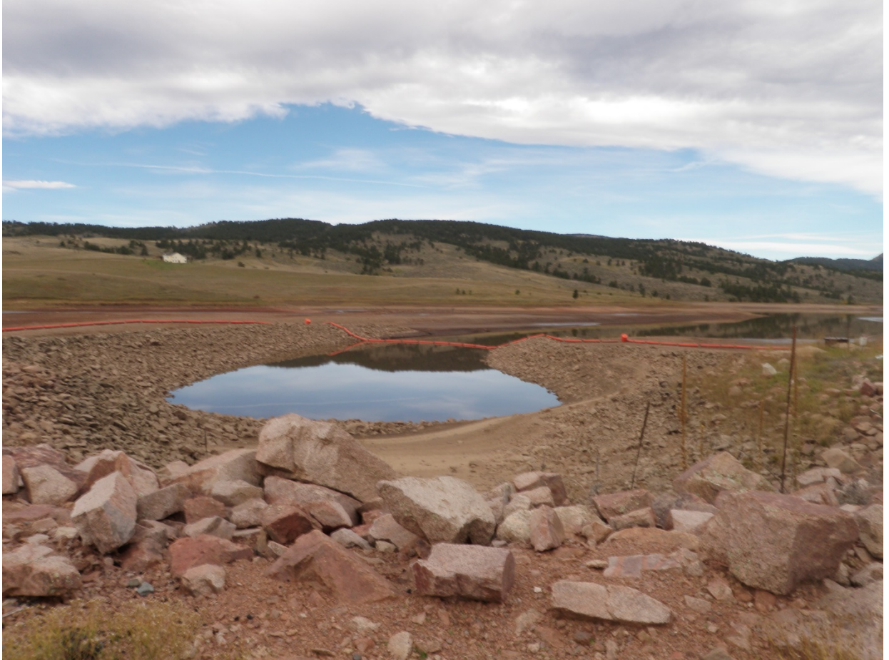
Figure 2 - Intake to Bald Mountain Pressure Tunnel to the Flatiron Powerplant with reservoir drawdown about 20 feet below normal full pool elevation 6,580.
