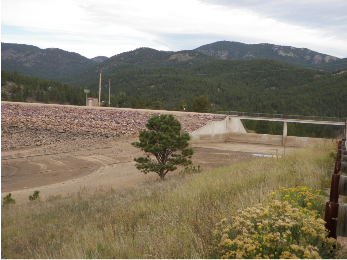
Figure 3 - Rattlesnake Dam and spillway with reservoir drawdown about 20 feet.
